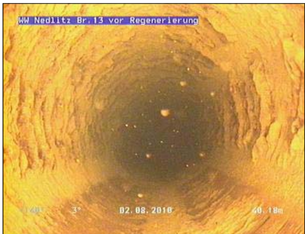
Photos: Well winding wire and PVC filter before and after completed regeneration using the hydropuls® process (source: pigadi)
